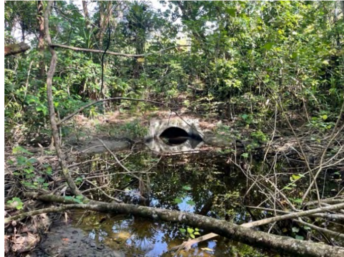
Photo 30. Culvert located south of airport near main road on the edge of the Galil mangrove.
