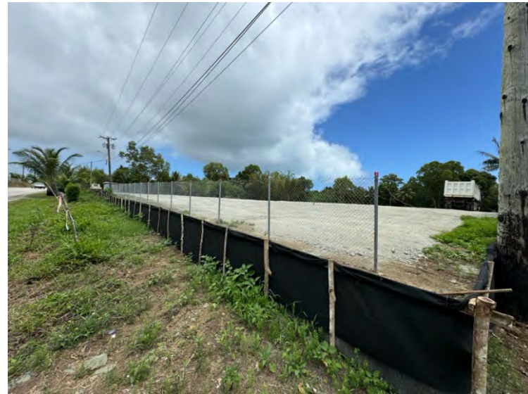
Photo 62. Construction staging area east of airport.
