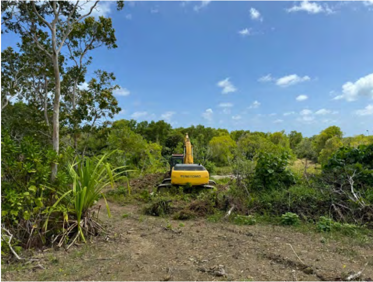
Photo 57. Active vegetation clearing east of airport.
