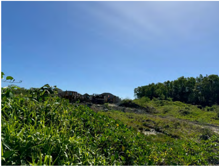
Photo 61. Construction area east of airport.
