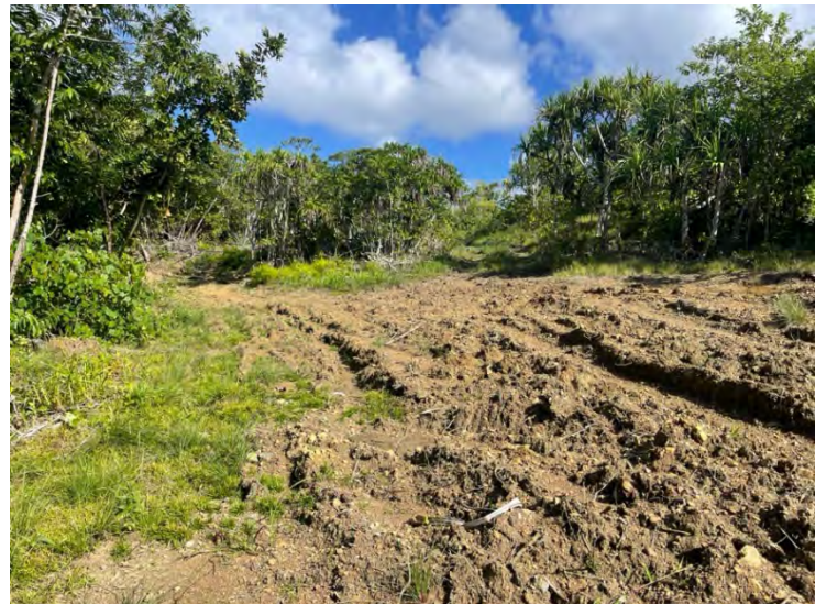
Photo 60. Cleared road east of airport.
