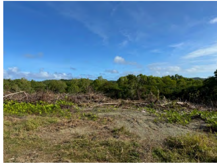
Photo 54. Cleared vegetation east of airport.
